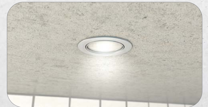
6. Install any built-in devices such as luminaires or loudspeakers.
