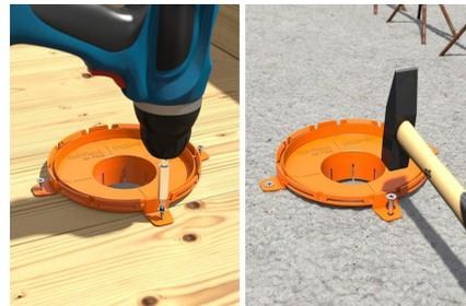
Fasten Uni-Flexx with screws or mounting brackets.
