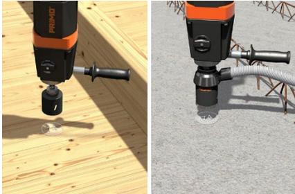
Drill 74 mm hole in exposed formwork or in filigree ceiling.
