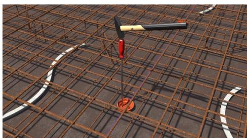
If the second reinforcement has already been attached, the front part can be positioned and nailed with the Primo nailer.
