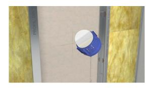
Stick the adhesive disk (P005) onto the lower part and remove the protective film.
