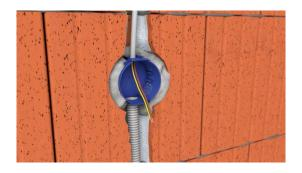
Mill the drill hole for the base of the box. Set the bottom part of the box flush, insert the cables and pipes.
