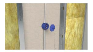
Attach the drill cover (P003) and insert the insulating wool.
