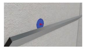
Plaster the wall and press the upper part in flush.
