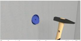
Break out the cover with a hammer and install the built-in appliance/socket.
