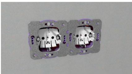
Fasten the device using the integrated screws.
