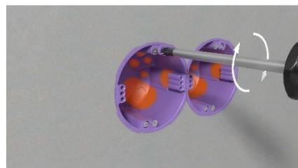
Insert the boxes into the drilled holes and tighten the screws.
